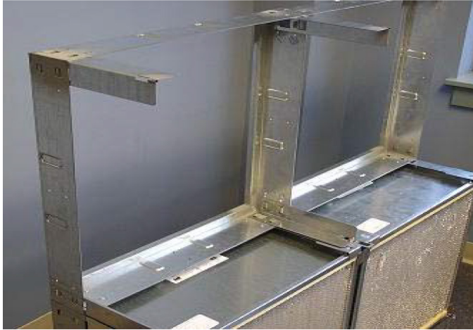
Figure 43: Insert HEPA Filter into Frame, until the Gasket Comes in Contact with the Holding Frame
